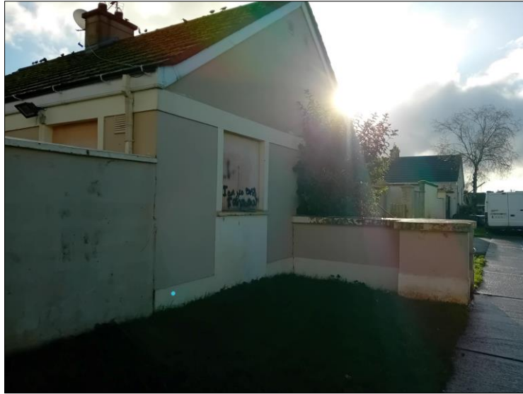
FIGURE 6. BUILDINGS AND ARTIFICIAL SURFACES (BL3)
